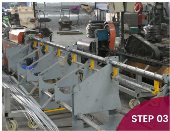
Wire Mesh Welding
