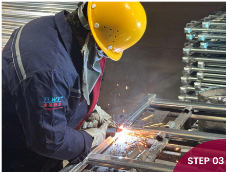
Steel Picket Fence Panel Welding
