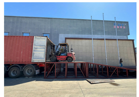
STEEL FENCE DELIVERY
