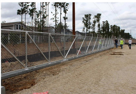
Chain Link Fence Suspended Gate
