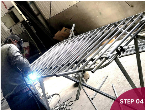
Crowd Control Panel Welding
