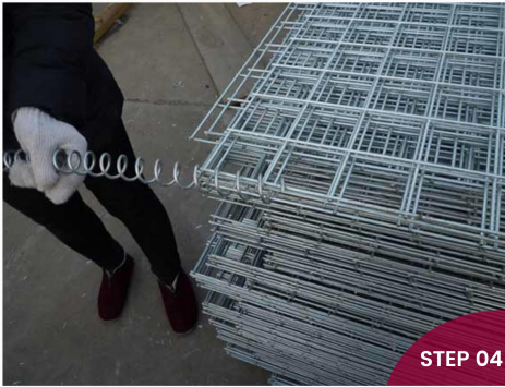
Adding Reinforcing Ribs
