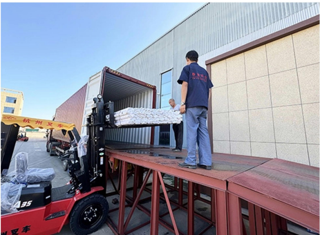
CHAIN LINK FENCE DELIVERY
