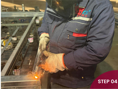
Square Tube Welding
