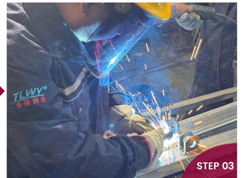
Steel Picket Fence Panel Welding
