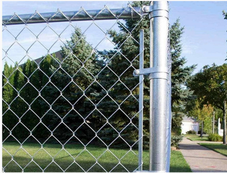
Tension Bar Assembly
