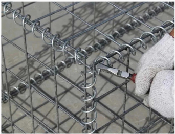
2.Welded Wire Mesh Panels Assembled With Spirals
