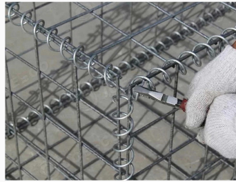
2. Welded Wire Mesh Panels Assembled With Spirals
